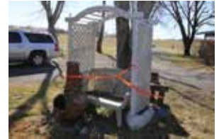
56. Chimney, Bench Etc
